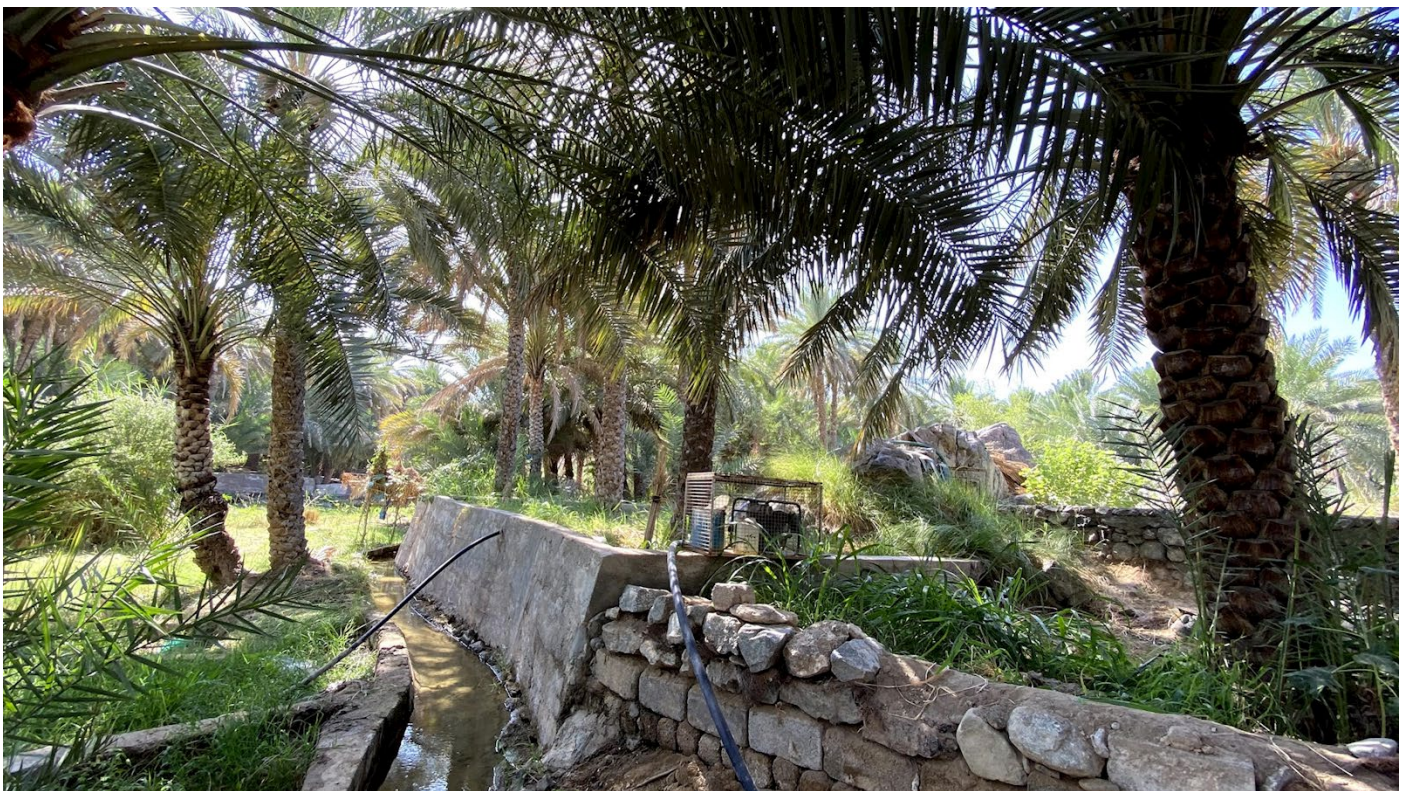
Traditional date palm farms usually irrigated with falaj system where water is channelled from underground wells to the farms.
