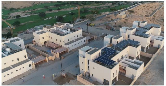
Figure 6: PDO's Awaifi Villas solar PV pilot awarded to two SMEs as nominated subcontractors to the primary EPC contractor. Solar pergolas deployed on the right-hand side villas were designed, constructed and commissioned by HTC.
